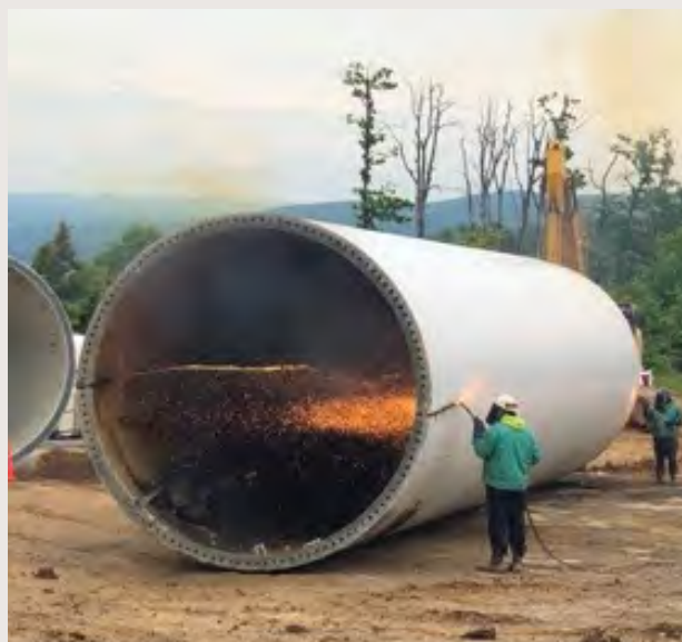
Workers cut sections of the old towers removed from Pinnacle Wind to prepare them to be recycled.
